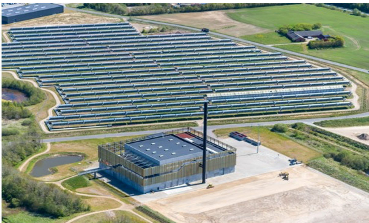
Figure 2: Brønderslev Biomass CHP plant and solar thermal field, Denmark (Source: niras.com, Case study details in: IEA TNCG, 2025)
