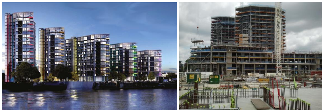
Figure 5.5: Artist impression Riverlight project and impression construction site in 2013 (picture IFTech)
