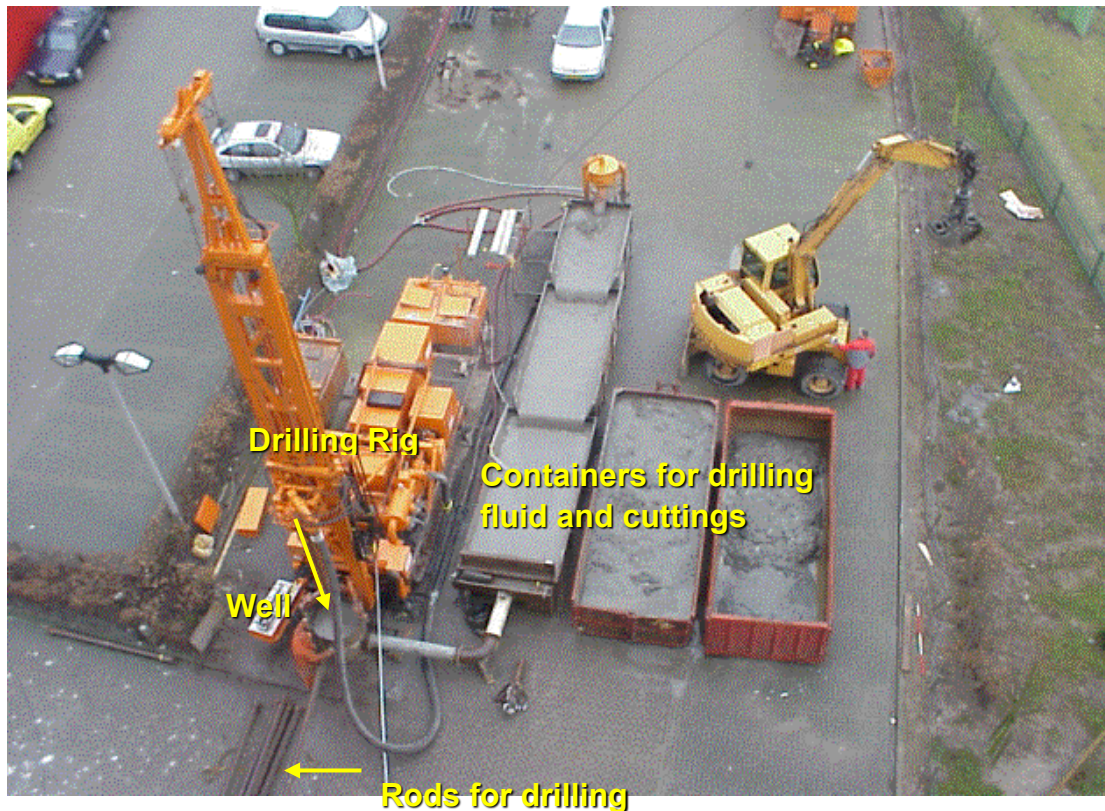
Figure 3.13: Overview well drilling site (IF Technology)
