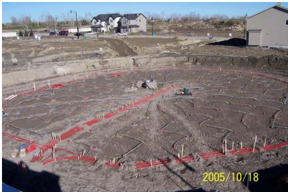
Figure 2.6: Drake Landing borehole field under construction and currently, as a landscaped park (NRCan)
