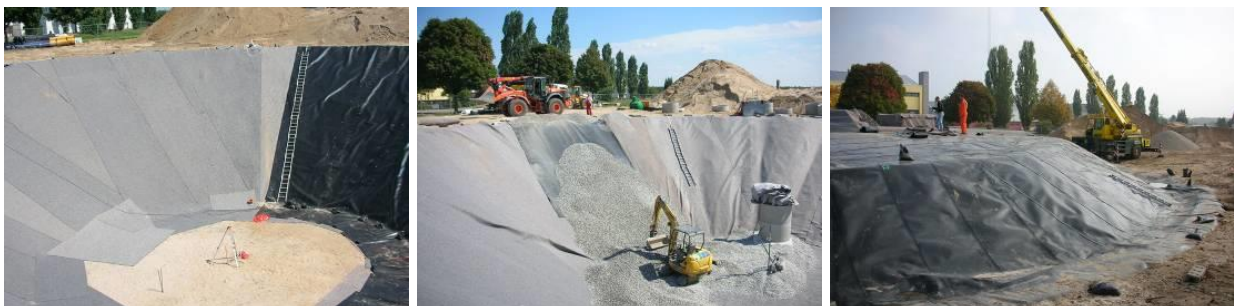
Figure 5.12: Construction phases of the PTES (Solites)
