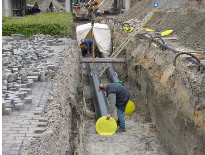
Figure 5.1 – Construction of main distribution loop (Eindhoven University)
