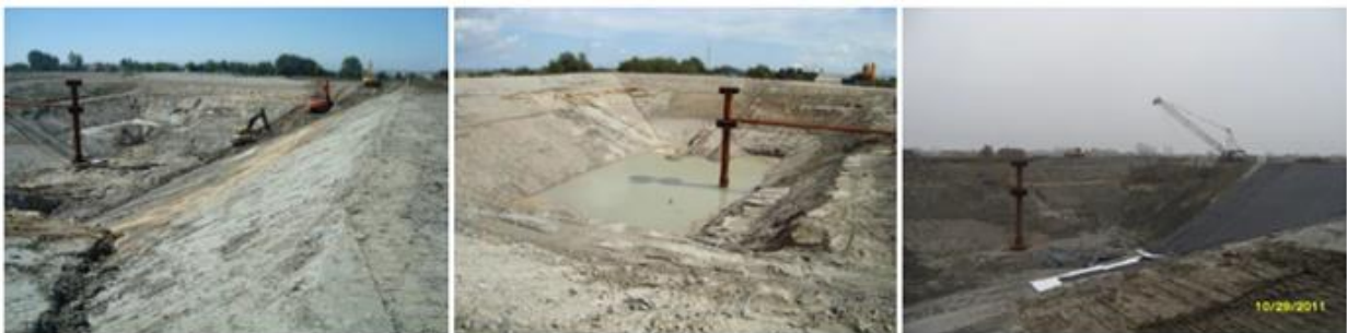
Figure 5.8: Pictures of the excavation process (PlanEnergi)
