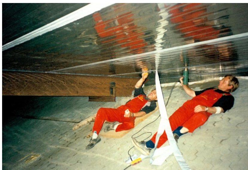
Figure 4.3. Mounting of cold store elements in Ottrupgård (PlanEnergi)
