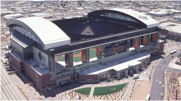
Chase Field, home of the Arizona Diamondbacks and location of a chiller plant. Photo by NRG.
