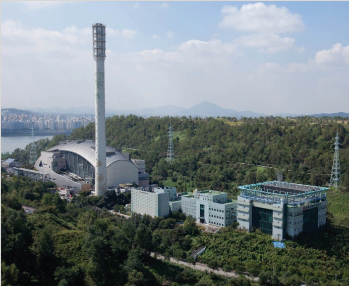
Sangam Integrated District Heating Plant. Photo by Taeyoon Yoon.
