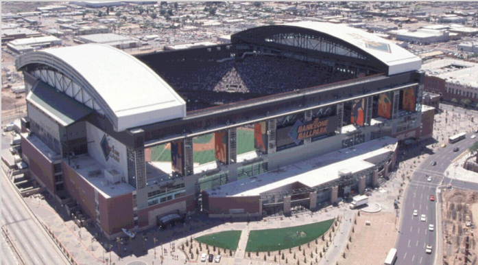
Chase Field, home of the Arizona Diamondbacks and location of a chiller plant. Photo by NRG.
