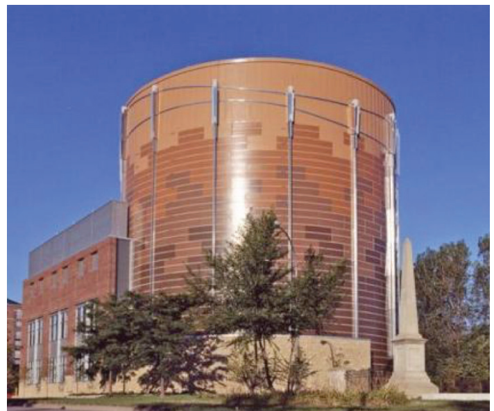
Thermal energy storage tank, District Energy St. Paul. Photo by Ever-Green Energy.
