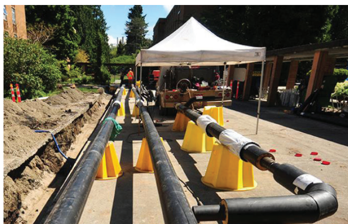
Hot water pipe installation at University of British Columbia. Photo by UBC.
