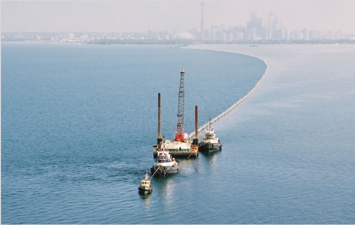
Intake pipes being deployed in Lake Ontario. Photo by Enwave Toronto.
