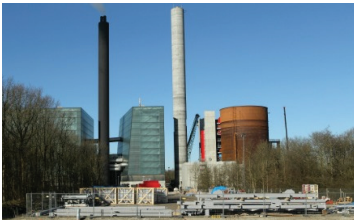
The new Lisbjerg biomass-fueled CHP plant, ready for commissioning. Photo by Aarhus Kommune.
