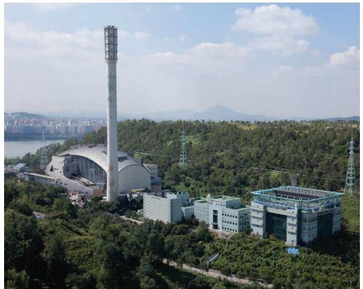
Sangam Integrated District Heating Plant. Photo by Taeyoon Yoon.
