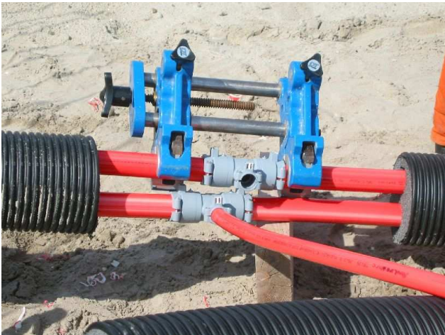
Fig.3. Example of welding the PB pipes
