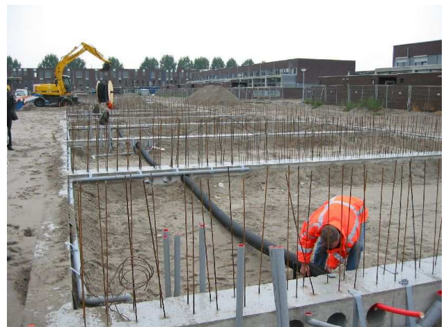
Fig.2. Installation of plastic pipes still requires some experience
