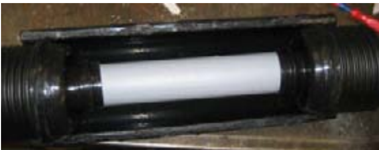
Figure 4.3: An open view of a wedge joint
