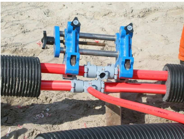
Fig.3. Example of welding the PB pipes
