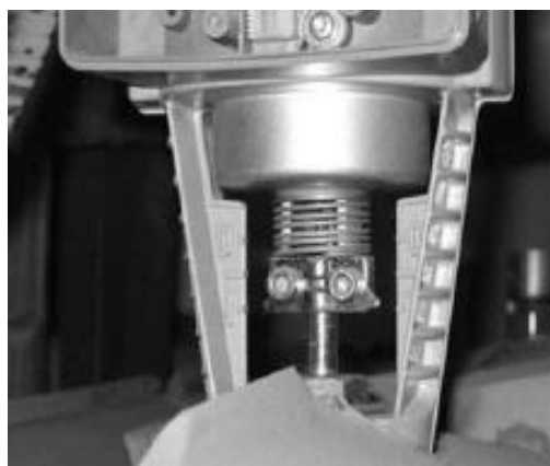
Figure 4.1-11: The connection between valve stem and actuator
