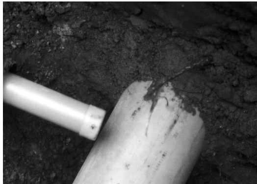
Fig. 4-18: Bedding of the pipeline in hydraulic drilling top: excavated gas pipe, bottom: schematic diagram [25]
