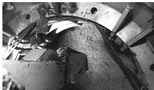
Fig. 4-25: Pipe propulsion for district heat transport pipeline (Line Mannheim-Heidelberg)
