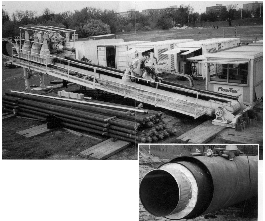
Fig. 4-17: Large horizontal hydraulic drill
