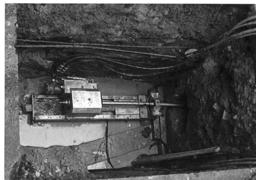
a) pilot pipe propulsion
