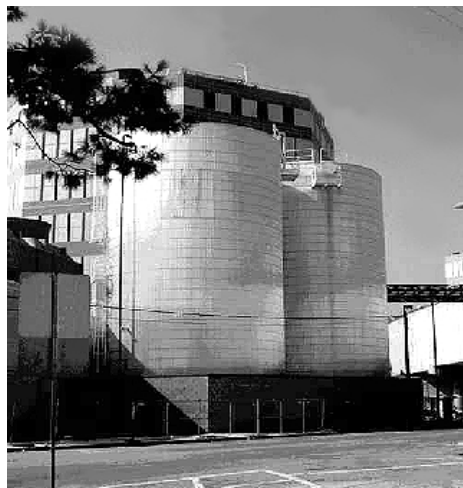
Figure 24 Atmospheric tank (Source: Cryogel)
