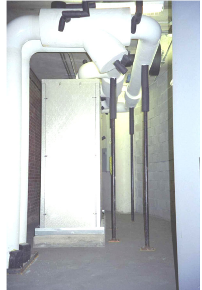
Part I Figure 7.3: ETS after installation
