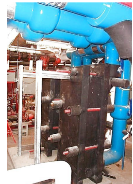
Part I Figure 4.4: Typical ETS for indirect connection
