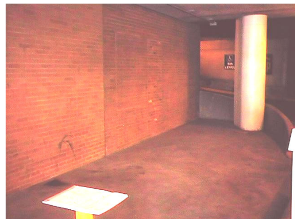
Part I Figure 7.2: ETS location before installation
