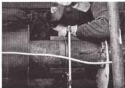
Fig. 5-3: The laying of Twin-Pipes Left: Welding Right: Parts
