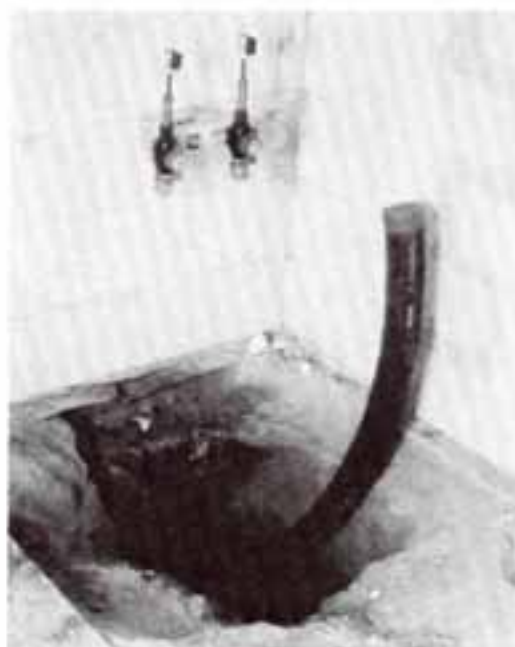
Figure 2.6: Assembly of house connecting fittings - joints prepared for the leakage test.
