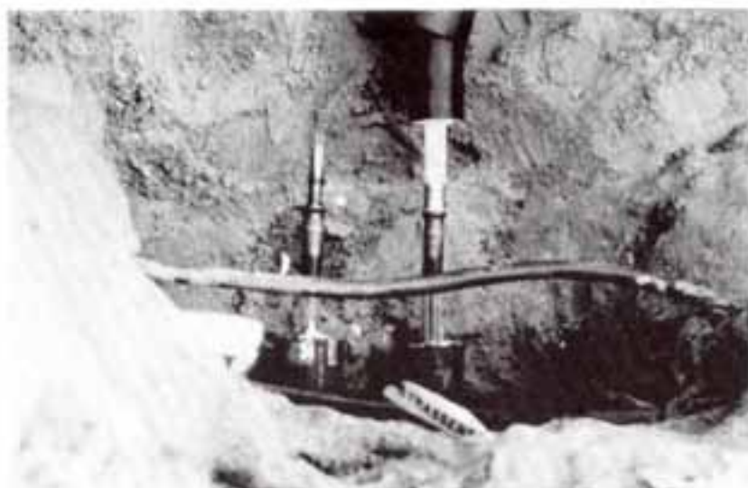
Figure 2.20: Assembly of the PEX/FLEX system.
