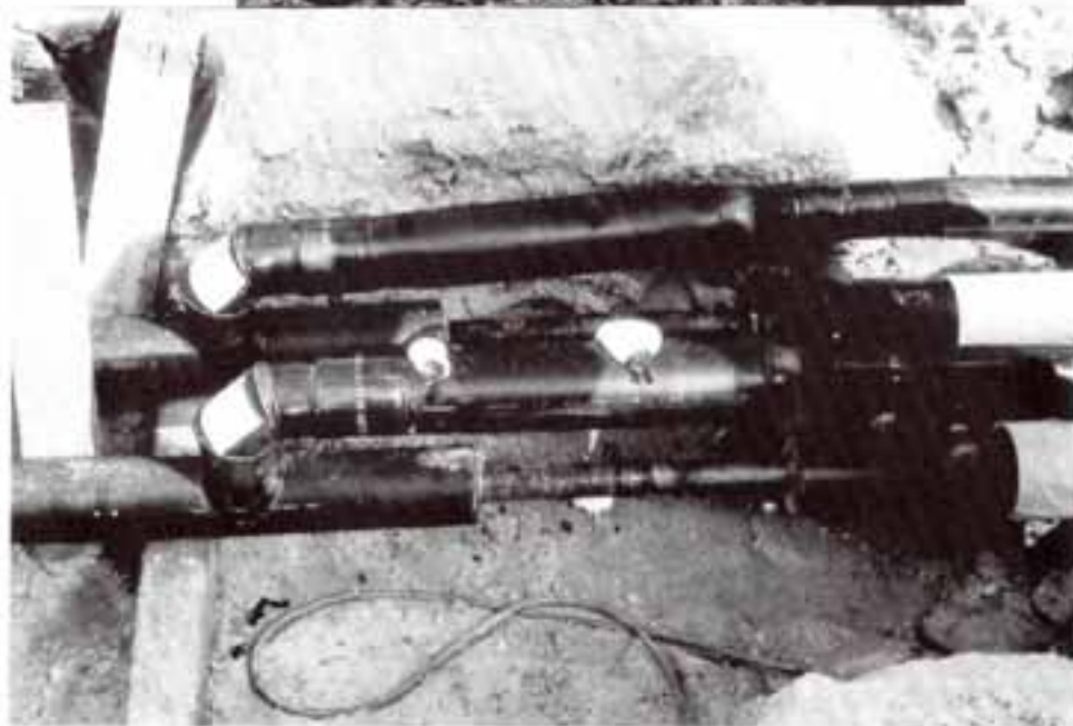
Figure 3.9: T-junction and parallel branch of plastic medium pipes to preinsulated pipes.
