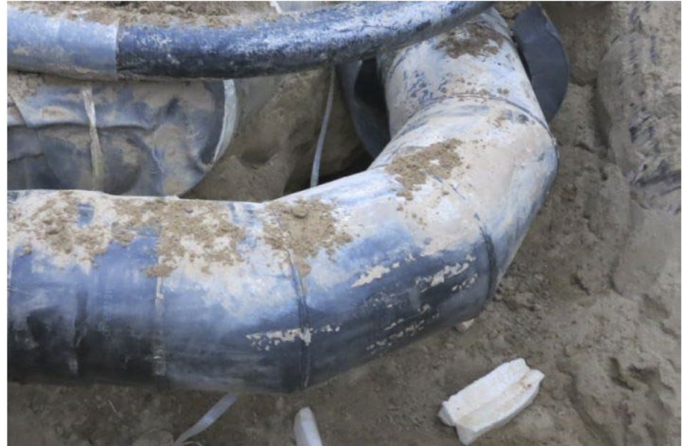
Investigation in a DH network 2017, source: EVN & AGFW
