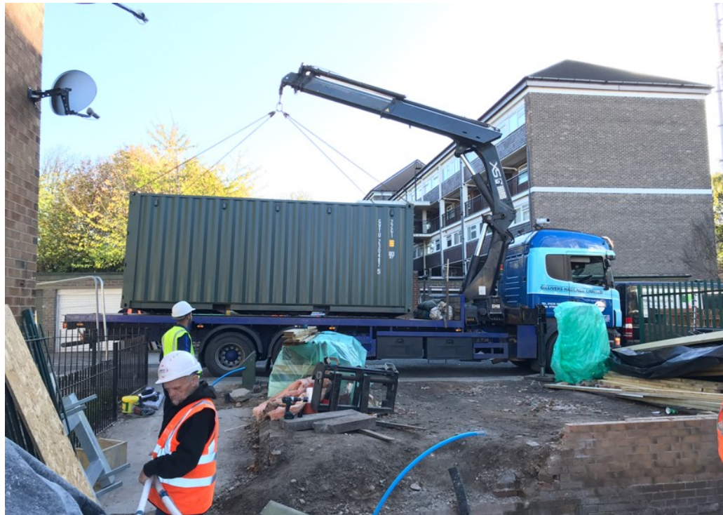
Energy Centre - installation
