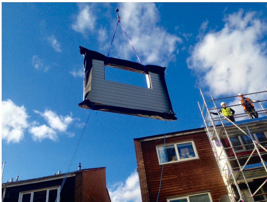
Installation of insulation panels
