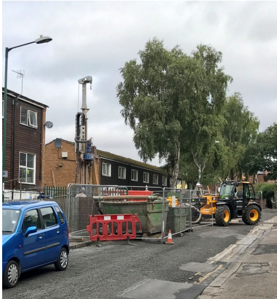
Bore Holes drilling (5 x 135m)
