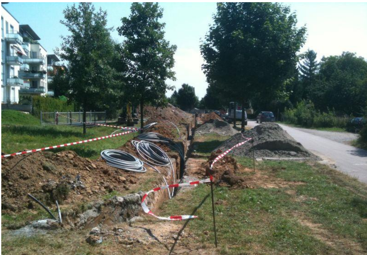
Figure 8. Trenches being built in the Sonnenberg district of Ludwigsburg.
