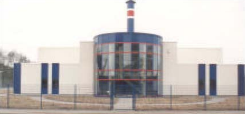
Geothermal heating plant Neustadt-Glewe photo O. Joswig
