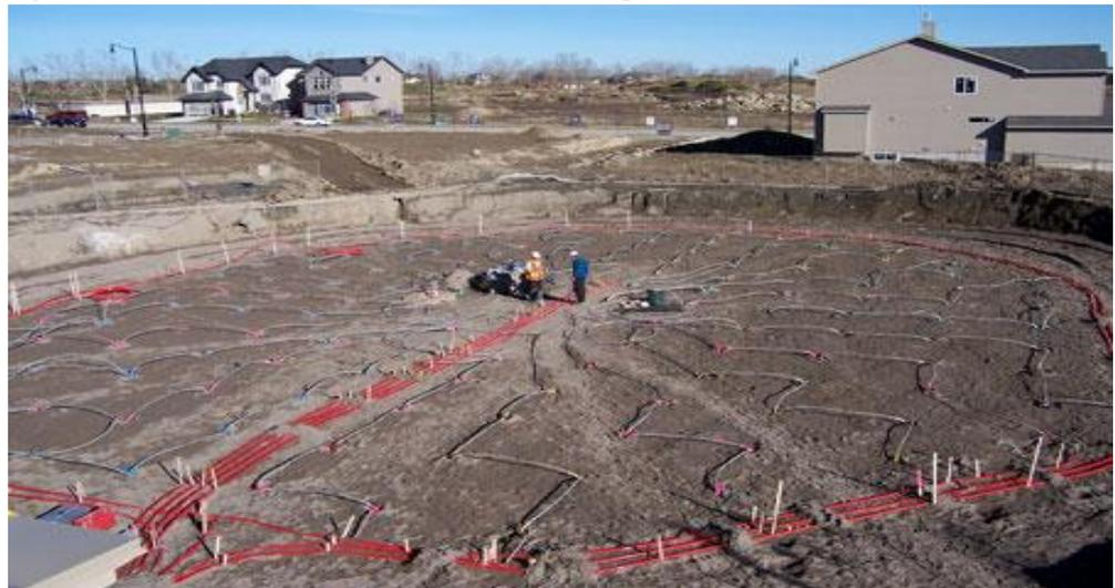
Figure 46: Excavation for the Boreholes at Okotoks
