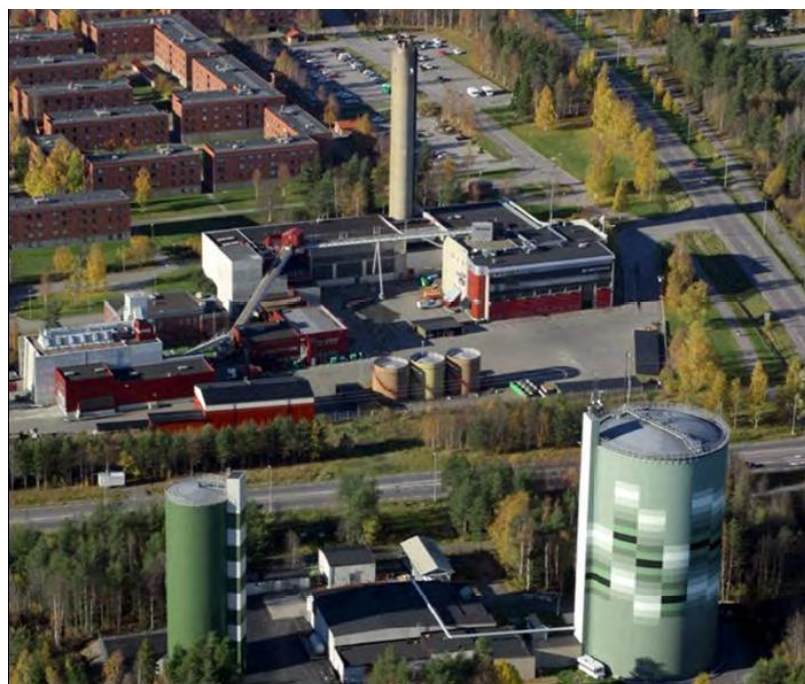
Figure 117. The Ålidhem plant, located in the central Umeå, Sweden, has 2 biomass boilers (25/35 MW) and two heat pumps using industrial waste heat (15/20 MW). It also has accumulators storing district heating and district cooling.
