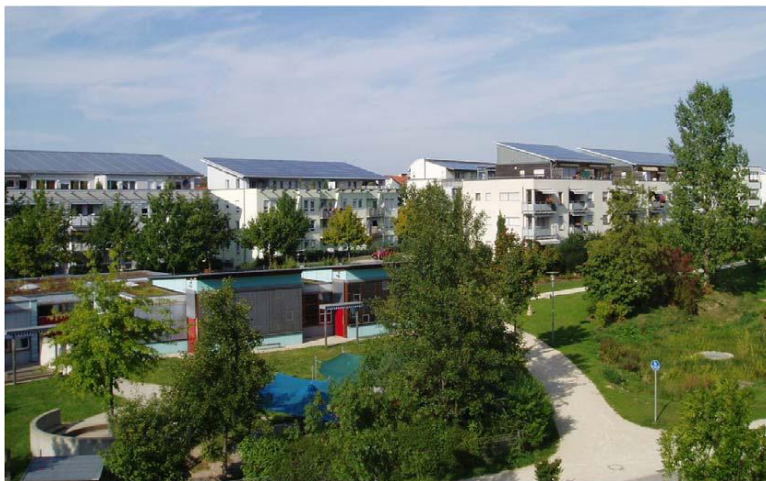
Figure 122. Solar block-heating Neckarsulm, Germany. Dalenbäck (2010).
