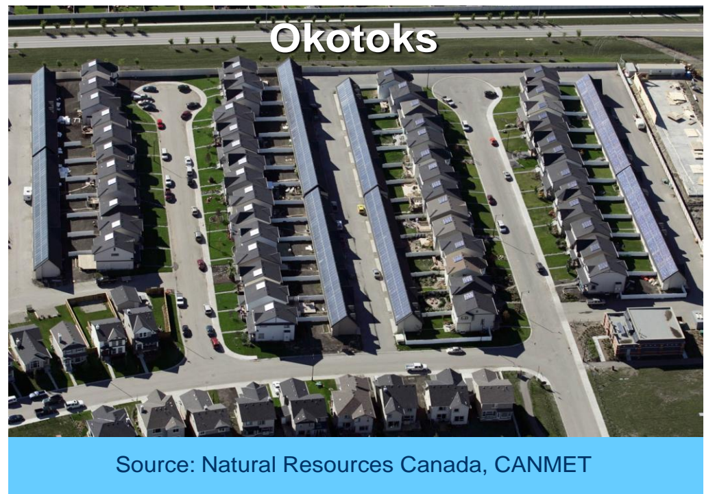
Figure 1: 52 Low-Energy Houses in the Drake Landing Solar Community, in Okotoks
