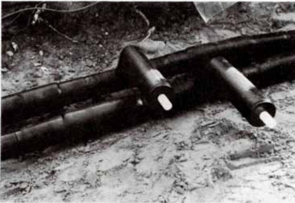
Fig. 3.3-3 Branch with Manufactured Tees
