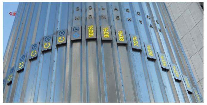
Figure 80. An LED visualisation on the buffer tank informs all passers-by how much thermal energy and how much electricity is currently produced by the sun and how much of the demand has been supplied in the last 24 hours (© SIR StrassI).
